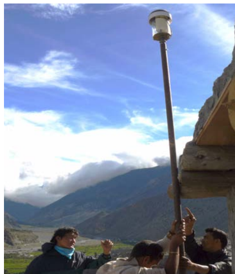
Deployment of a community-based Hybrid Wireless Network using TV white space and Wi-Fi spectrum in remote valleys around Manaslu Himalaya in Nepal. Photo credit: APNIC
